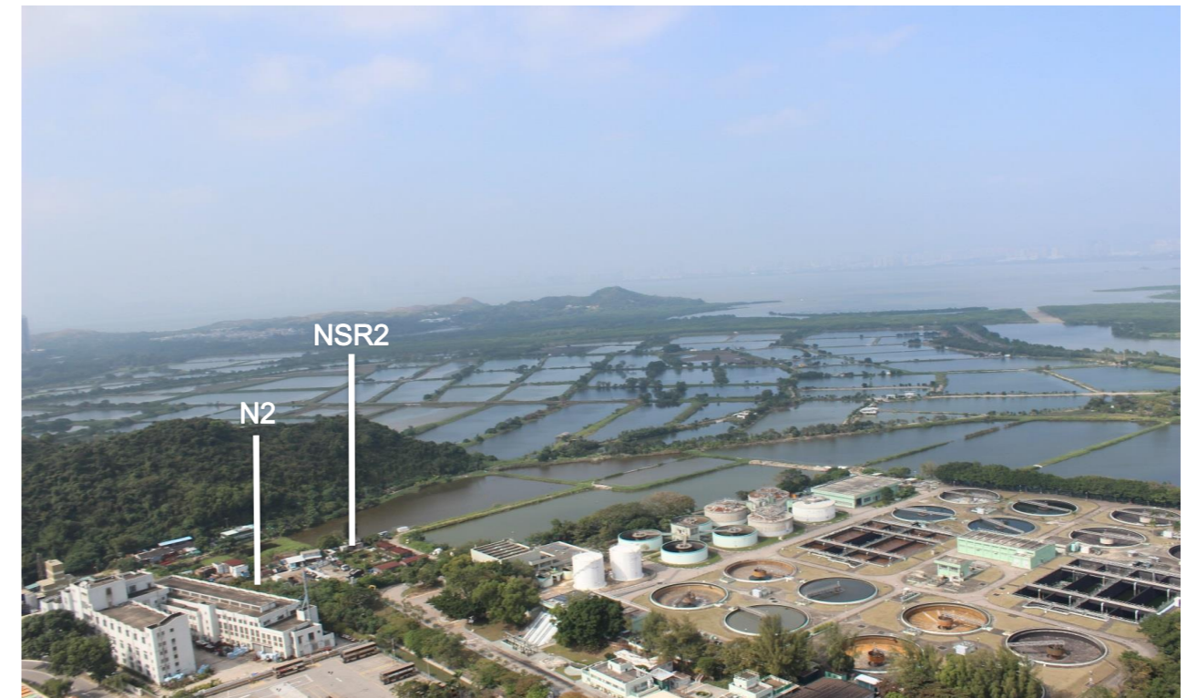
NSR2 Squatter house at the west of Yuen Long STW
